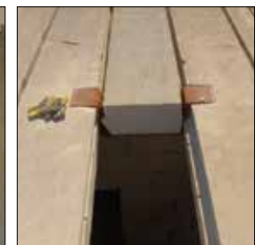
A/C Opening with Clamping
